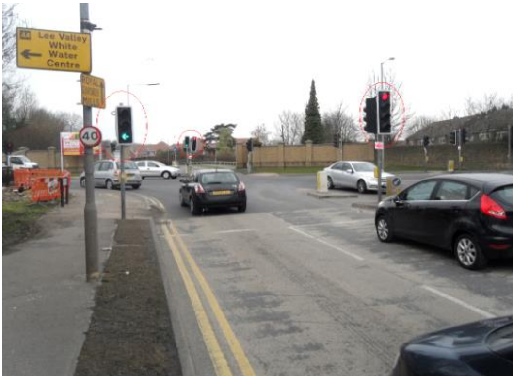
Figure 2: Meridian Way left turn traffic is at green at the same time as Station Way traffic. Note that signal for the ahead/right turn lane is still at red and drivers wishing to proceed ahead to Beaulieu Drive must wait for the green signal.
