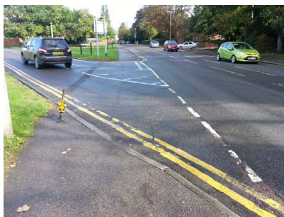
Photographs: Looking northeastbound on B1393 High Street
