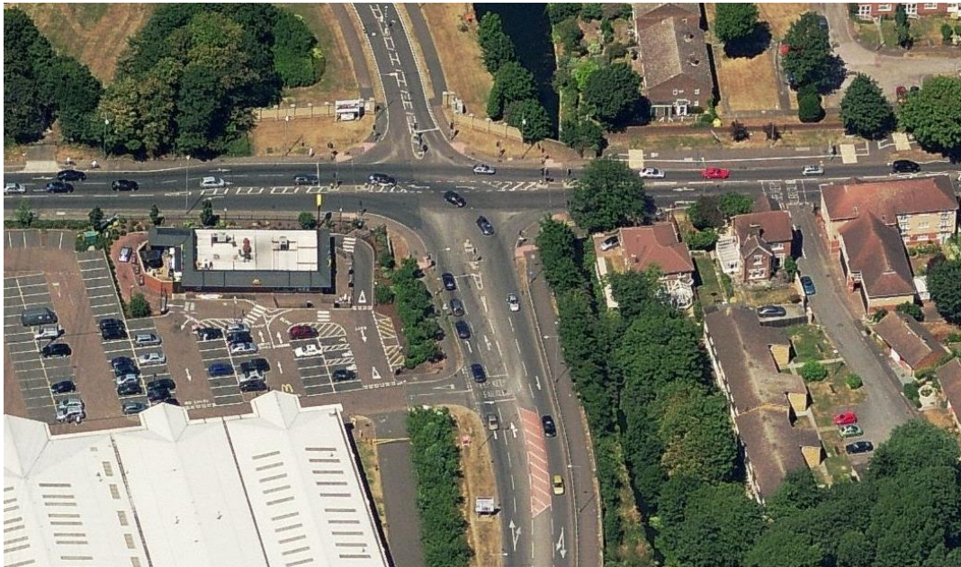
Figure 1: Aerial photograph of the junction. A121 Meridian Way approach is in the foreground
