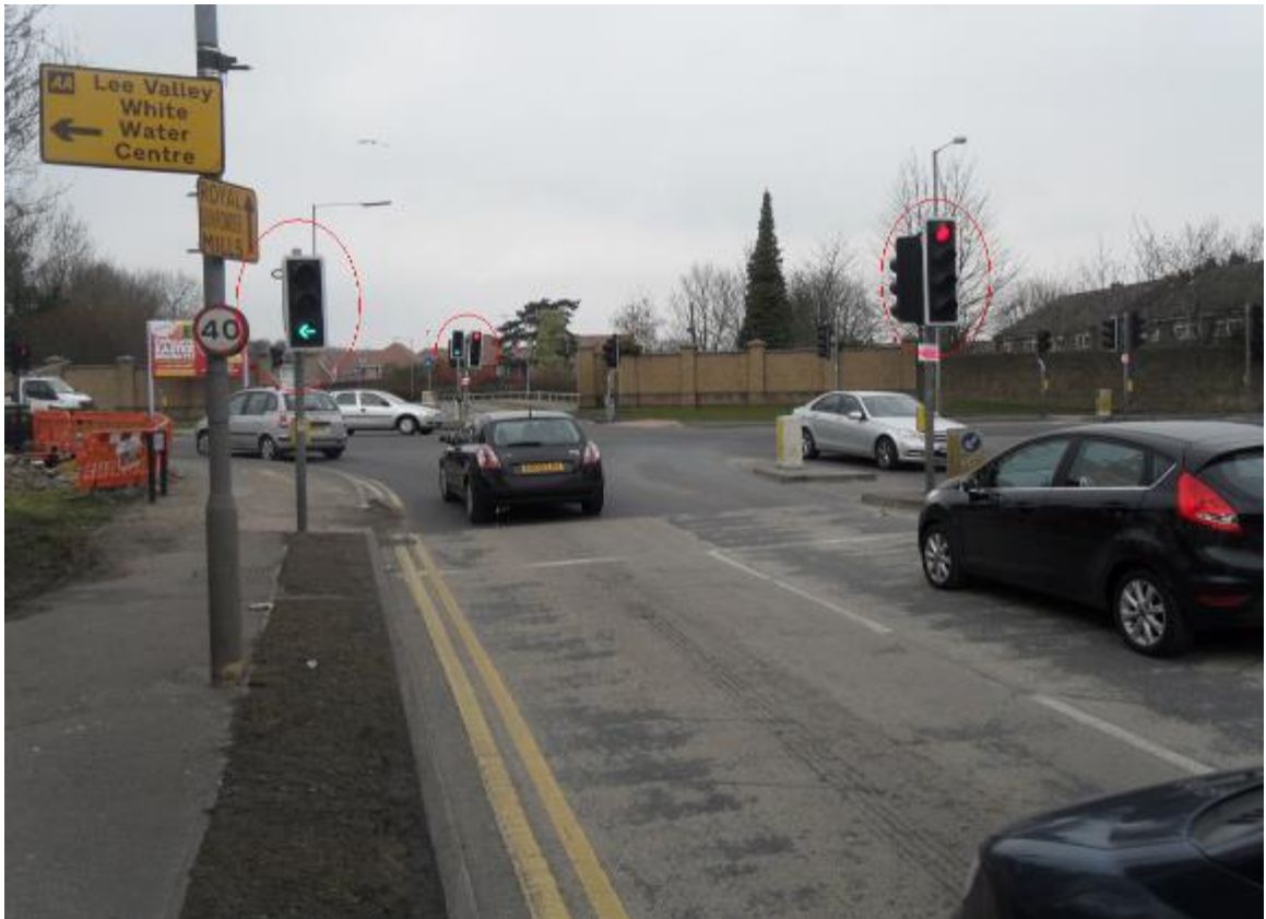
Photo 2 – Different traffic signals relate to the nearside and offside traffic lanes.
