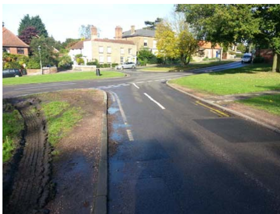
Photographs: Looking north westbound on Lindsey Street link road
